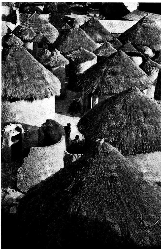
Houses of the Senufo tribe, Ivory Coast. The cylindrical walls are made of mud, the conical roofs of thatched grass
