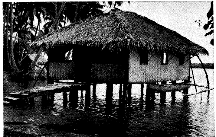
Polynesian pile dwelling of frame construction with lattice-work siding of coconut fibres and thatched roof drawn in a gable; Raiatea Island, Society Islands
