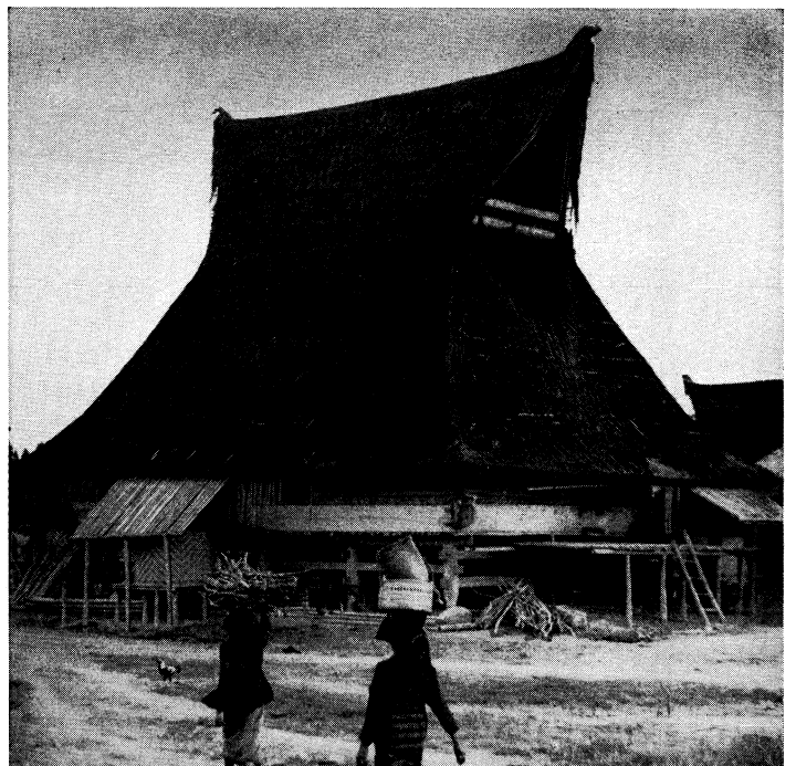
Low-walled house of frame construction, slightly elevated from the ground, with a high horned roof, a communal dwelling of the Bataks in western Sumatra
