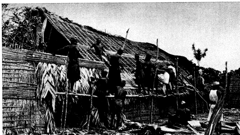
Kuba (Bushongo) tribesmen building a rectangular gable-roofed house out of palm thatch in the lower region of the Congo river, Republic of the Congo
