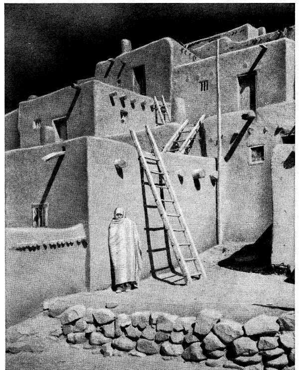
Pueblo of the Taos Indians, New Mexico. The square rooms are made of adobe and set one upon the other to form a pyramid, with ladders used to reach the upper levels
