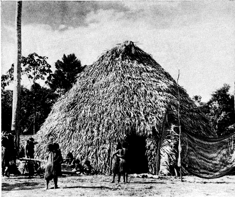
Oval community house of the Yagua tribe of northeastern Peru. Sections of plaited palm leaves are tied to a lashed-pole framework. Palm screen at right serves as the door
