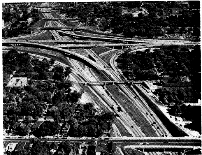
Expressway interchange where the Lodge and Ford expressways meet. Five levels separate the traffic lanes and permit transfer from one expressway to another
