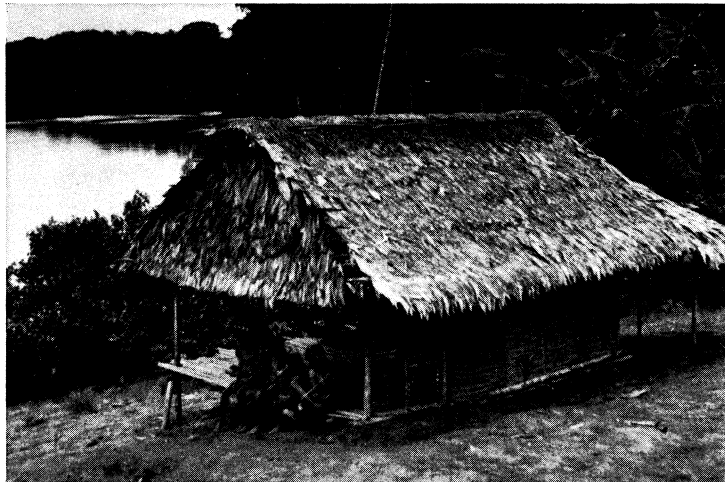
Hut of the Oyampi Indians on a bank of the Oyapock river, French Guiana. The structure is basically a platform with a gabled roof and one wall serving as a windbreak
