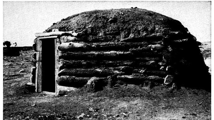
Hogan of the Navahos, a nomadic tribe of the southwest. Dirt heaped on the roof and used as chinking between the logs made the dwelling rainproof
