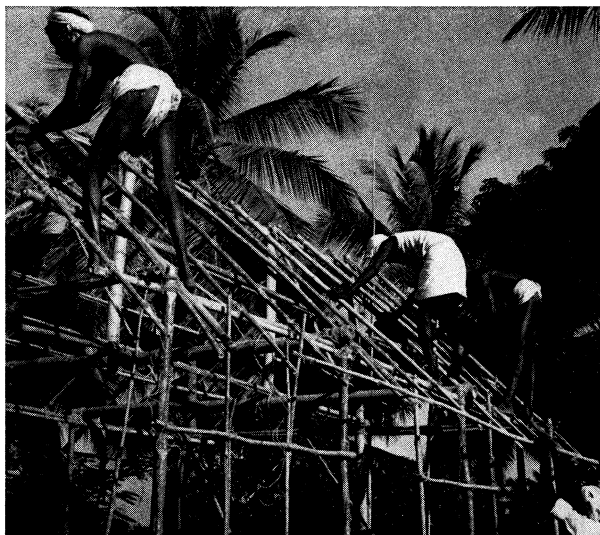
Tribesmen of India building a rectangular gable-roofed house, the frame of which is made of bamboo poles lashed together with vine ropes
