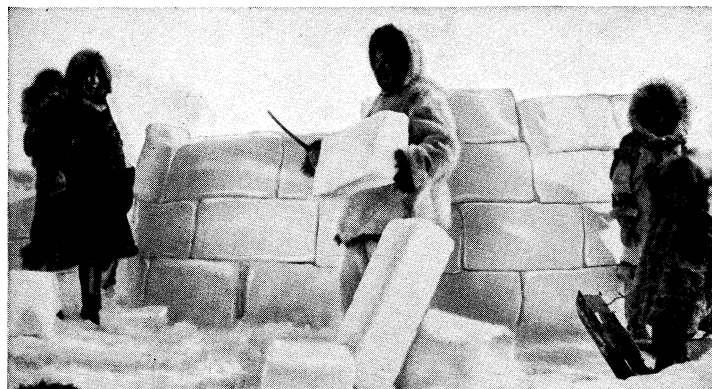
Alaskan Eskimos building an igloo with carved blocks of snow. The blocks are laid in an upward spiral to form a dome
