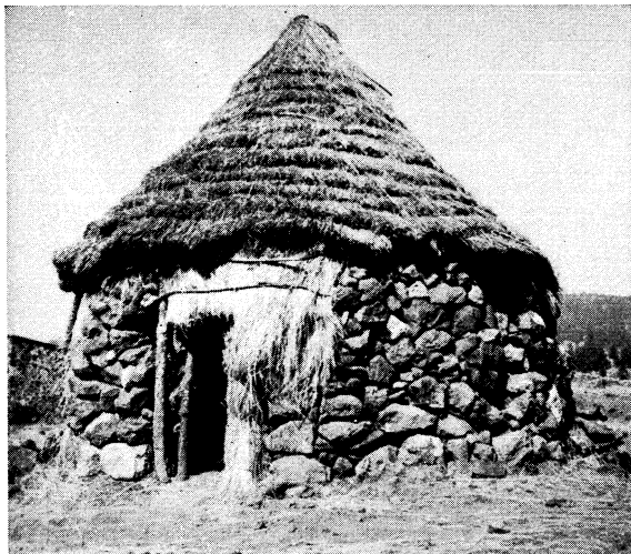
A round house of stones with a conical thatched roof, a typical dwelling of the Indians in the highlands of northern Mexico
