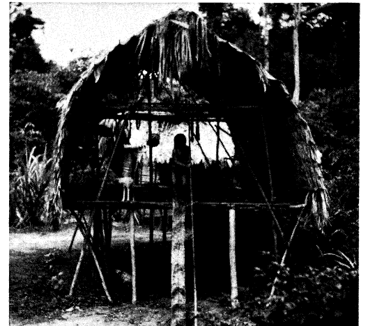
Another platform dwelling in the Amazon region of Brazil. Pilings serve as support for the flooring and as a frame for the roof. A notched tree is used as a ladder
