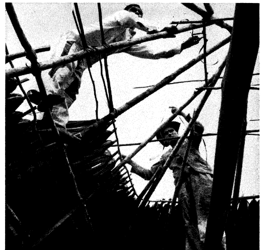
Lashing palm fronds to pole supports to make a thatched roof over a house in Colombia
