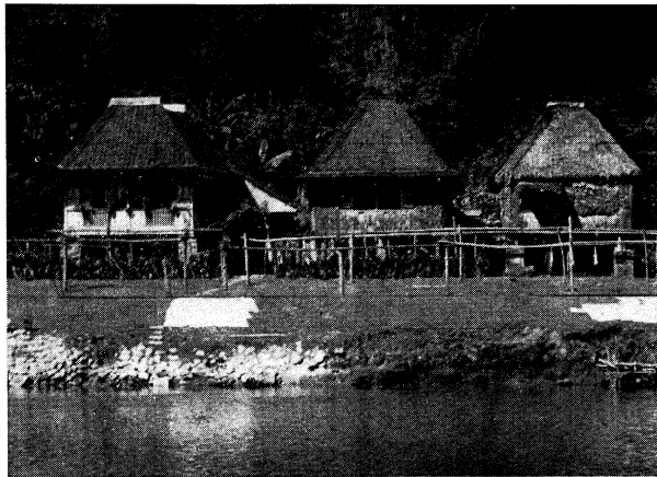
Pile dwellings of bamboo-frame construction with thatched roofs and siding, Luzon Island in the Philippines
