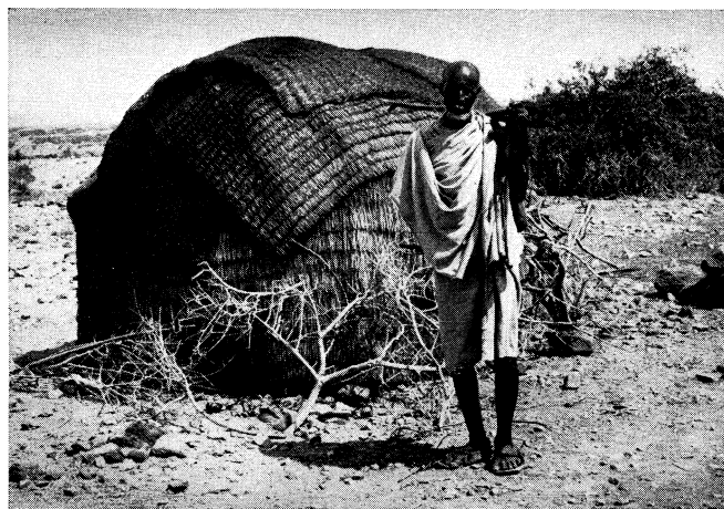
Shelter of the nomadic Isa tribe of Somalia, a portable, low-domed tent of reed mats supported by a hemispherical framework of curved poles
