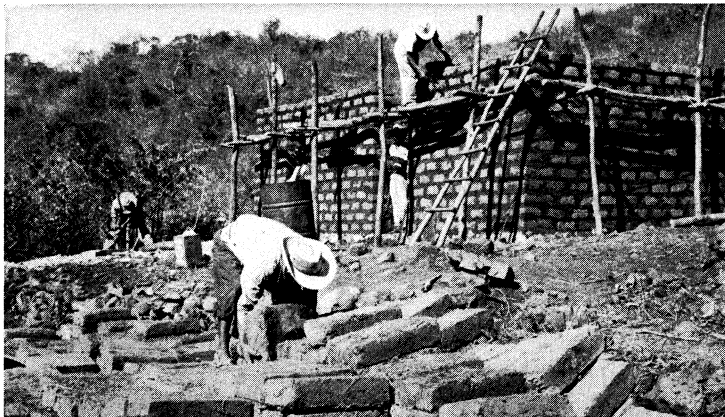
Construction of a house in Guatemala with adobe, sun-dried clay bricks, a principal building material of arid and semiarid regions throughout the world
