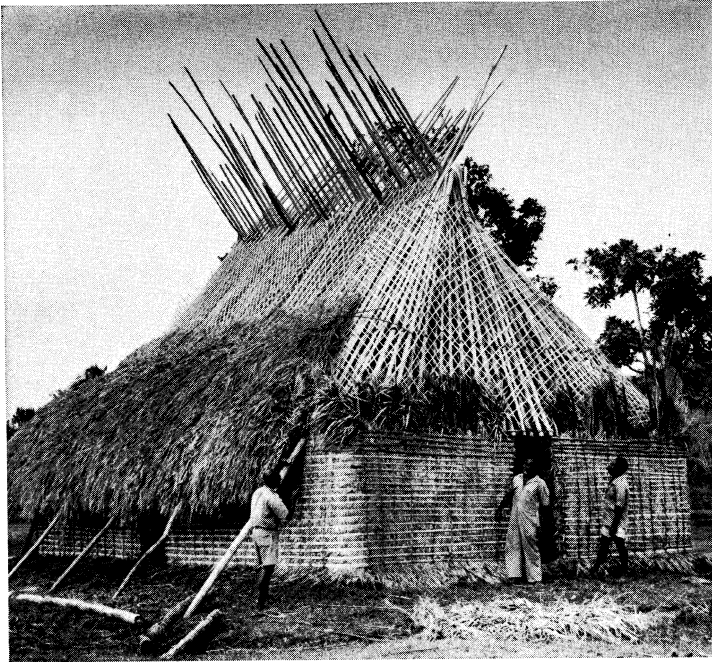
Fijians building a house of thatched reed leaves. The main support is heavy bush timber over which a framework of bamboos and reeds is laid and fastened by vines
